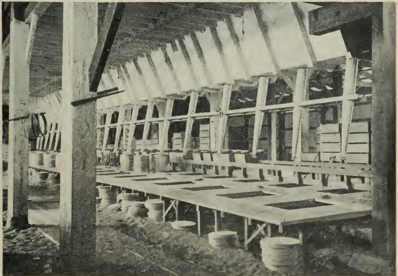
Fig. 11.—Arrangement of two packing houses for sawdust packing in kegs and drums. Note the solid construction of the benches, and the chutes for bringing the sawdust from the overhead storage bins to the packing benches.
